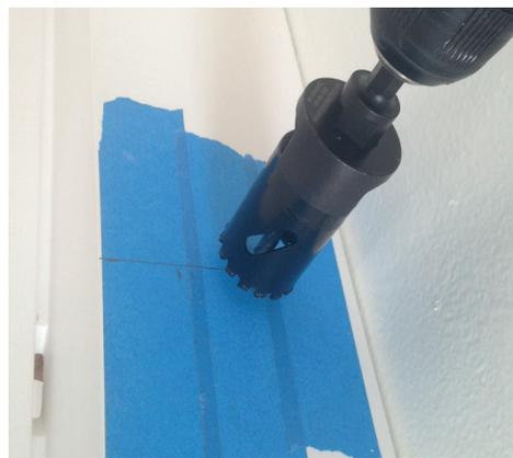
The drilling is done in two steps. First, drill a locator hole through the countertop at each of the three marks. This hole should be just slightly smaller than the size of the pilot bit of your carbide grit hole saw. Using these holes
