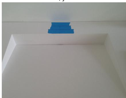
Lay the countertop/sink across a solid pair of sawhorses. Apply painters blue tape to the approximate area of where you want the faucet to go. Be generous in your tape coverage; however it is not necessary to apply multiple layers of tape. The purpose of the tape is to offer a little protection to the countertop and to give you a better surface to write on.
