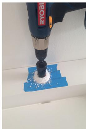
Keep the drill speed moderately low... just apply enough power to keep the holes saw cutting at an even rate. If the saw seems to be bogging down, increase the speed a little. Don't exert too much downward force... let the sharp hole saw do the work.
